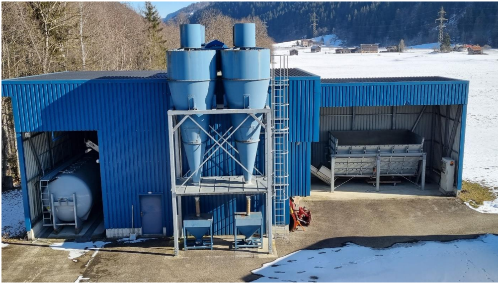
baghetg cun schigentera ad aria freida, seniester silo da transport dil gliet ella fabrica da cement
